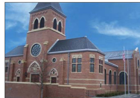
Institutional Category - Churches Sacred Heart Parish Church Weymouth, Massachusetts Architect: The S/L/A/M Collaborative Mason Contractor: Commercial Masonry Corporation Owner: Roman Catholic Archdiocese of Boston Engineer: The Collaborative Engineers Photography: The S/L/A/M Collaborative
