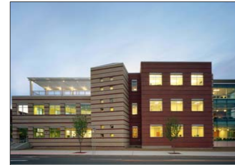
Best Contemporary Design Project - Brick & Stone Pfizer Clinical Research Unit New Haven, Connecticut Architect: The S/L/A/M Collaborative Mason Contractor: Lombardo Bros. Masonry, LLC Owner: Pfizer Corporation CM: Whiting-Turner Contracting Company Engineer: The S/L/A/M Collaborative Photography: Woodruff/Brown
