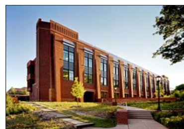
Educational Category - College Classrooms Yale Class of 1954 Chemistry Research Building New Haven, Connecticut Architect: Bohlin Cywinski Jackson Mason Contractor: NER Construction Management CM: William A. Berry & Son Owner: Yale University Engineer: Cannon Design Photography: Nic Lehoux Photography
