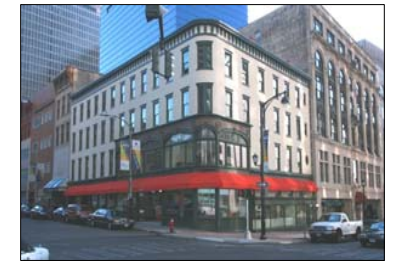
Restoration Category - Small Projects Stackpole Moore Tryon Building Hartford, Connecticut Architect: Maier Design Group, LLC Mason Contractor: Armani Restoration CM: Master's Construction Corporation Owner: Newgate Corporation Engineer: GM2 Associates Photography: Maier Design Group, LLC
