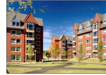
Educational Category - College Dormitories North Residential Apartments - UMASS Amherst, Massachusetts Architect: Architectural Resources Cambridge Mason Contractor: Chabot and Burnett CM: Dimeo Construction Company Owner: University of Massachusetts Amherst Engineer: LeMessurier Consultants Inc. Photography: Studio of Warren Patterson
