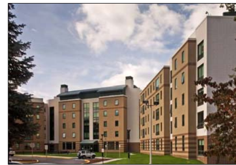
Best Sustainable Design Project New Residence Hall at Rhode Island College Providence, Rhode Island Architect: RGB Design Studio Mason Contractor: Costa Brothers Masonry Inc. CM: Bacon Construction Company Owner: Rhode Island College Engineer: Odeh Engineers, Inc. Photography: Focus Photography
