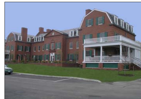
Best Structural Masonry & Design Project Flinn Hall & Edelman Hall Hotchkiss School - Lakeville, Connecticut Architect: Robert A M Stern Architects Mason Contractor: Lombardo Bros. Masonry, LLC CM: O & G Industries, Inc. Owner: Hotchkiss School Engineer: DeStefano Associates Photography: Hotchkiss School
