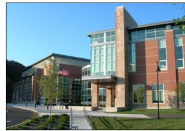
Educational Category - High Schools Swampscott High School Swampscott, Massachusetts Architect: SMMA Mason Contractor: Fred Salvucci Corporation CM: J & J Contractors, Inc. Owner: Town of Swampscott Engineer: SMMA Photography: SMMA
