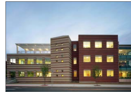
Best Contemporary Design Project - Brick & Stone Pfizer Clinical Research Unit New Haven, Connecticut Architect: The S/L/A/M Collaborative Mason Contractor: Lombardo Bros. Masonry, LLC Owner: Pfizer Corporation CM: Whiting-Turner Contracting Company Engineer: The S/L/A/M Collaborative Photography: Woodruff/Brown
