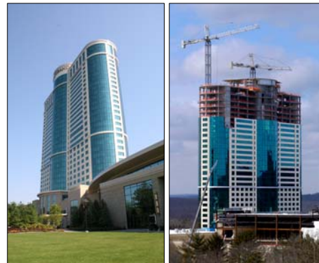
Special Award Project - Concrete Construction Foxwoods Casino MGM Grand Hotel Ledyard, Connecticut Manafort Brothers, Inc.
