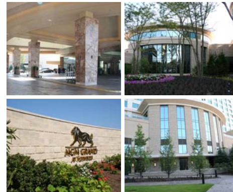
Special Award Project - Stone Masonry Foxwoods Casino MGM Grand Hotel Ledyard, Connecticut B.W. Dexter II, Inc.
