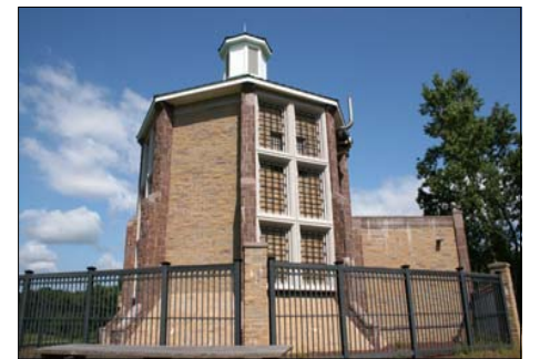
Commercial Category - Industrial Projects Fisher Meadows Well Pump House Avon, Connecticut Architect: Tuthill & Wells Architects Mason Contractor: John Filloramo Construction Company CM: Master's Construction Corporation Owner: Avon Water Company Engineer: Buck and Buck LLC, Engineers Photography: IMI
